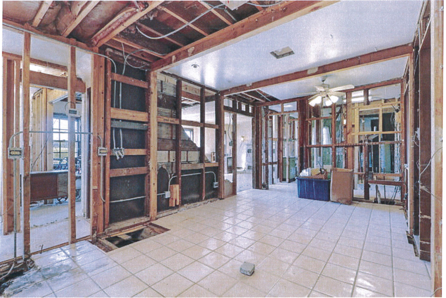
Gutted Interior of House Next Door – Listed for $279,900 ($147.47/sf)
