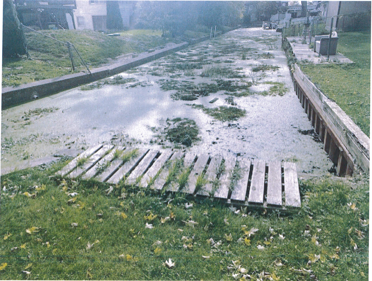
Appellant Comp #3 – Inferior narrow channel (25' wide)
